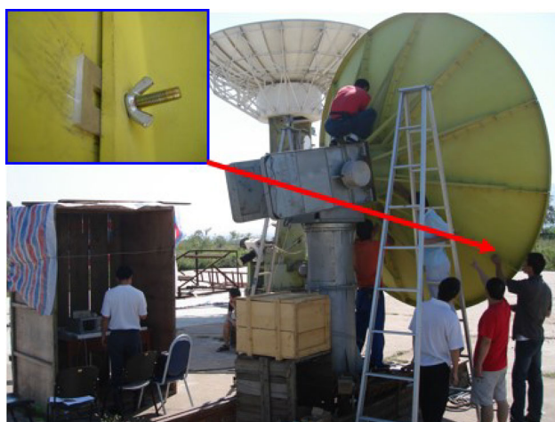
Fig. 6 Panel displacement by filling gaskets (back view)
