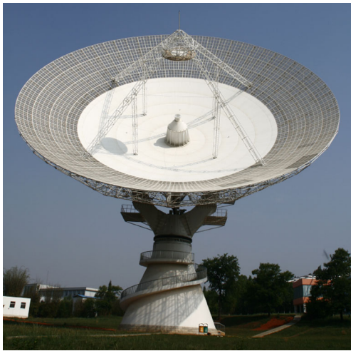
Fig. 1 S/X dual band reflector antenna with 40 m diameter, TT&C station located in Kunming for lunar exploration program
